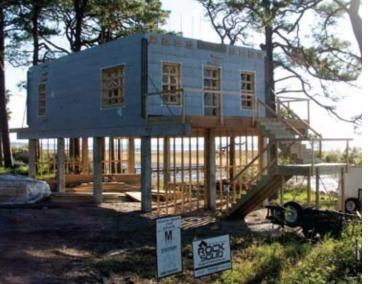
Rock Solid Construction builds frequently on the nearby coast, using insulated concrete forms that are reinforced with rebar and sandwiched between polystyrene panels. This home by Rock Solid went up off Highway 98 near Carrabelle. Photo courtesy
